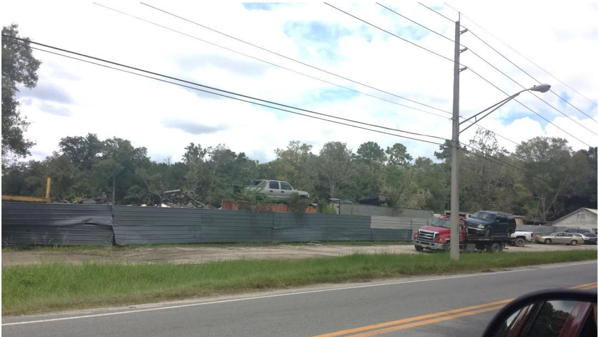
Figure 1. Subject property viewed looking north from Beaver Street showing existing vehicular use area.
